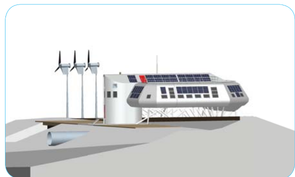
Figure 8: Look out for the pipe that forms the entrance to the garages as well as to the station itself.
